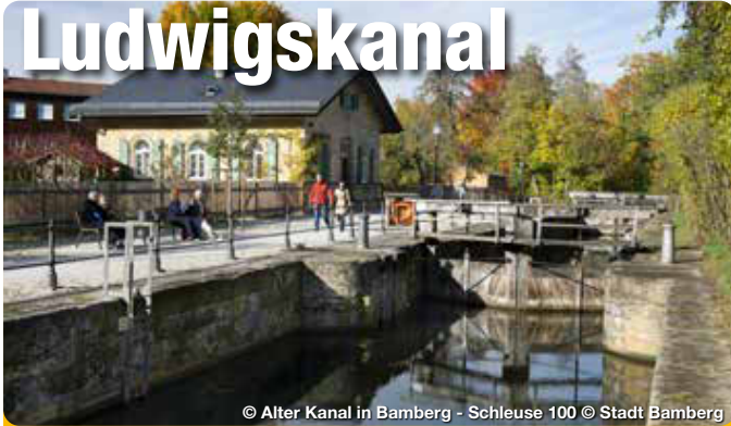
© Alter Kanal in Bamberg - Schleuse 100 © Stadt Bamberg
